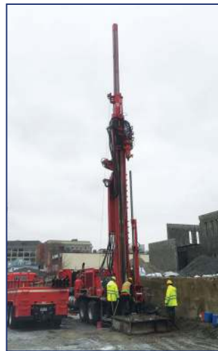
Ground source heat pump drilling.
